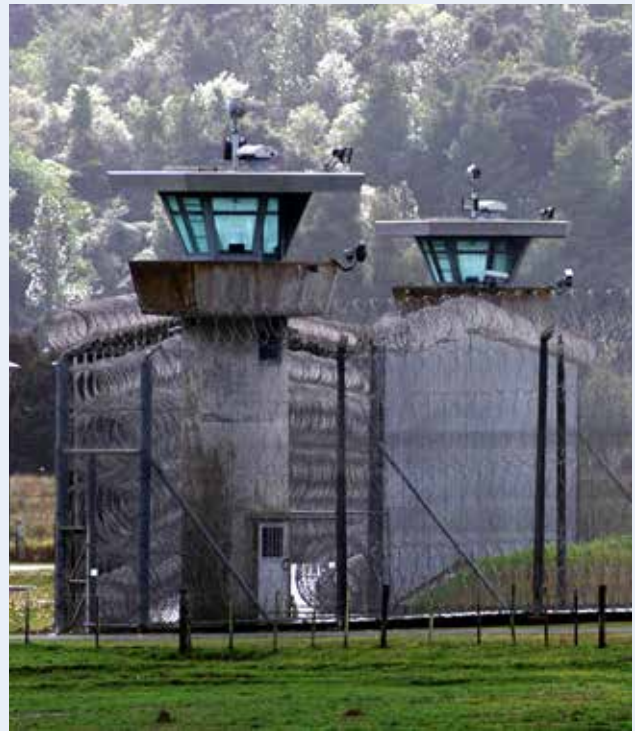
Paremoremo maximum-security prison, Auckland. New Zealand has one of the highest prison-population rates in the world.
